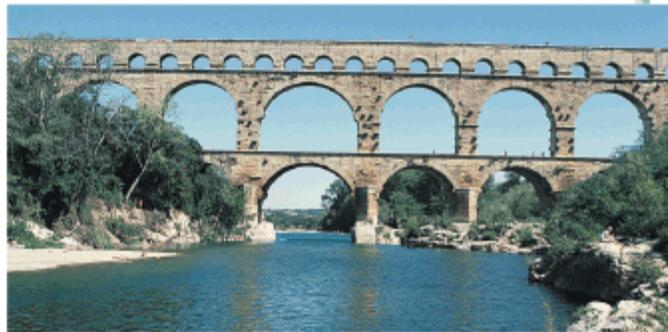
The arches in this Roman aqueduct, above the Gard River in France, are typical of arches you can find throughout regions that were once part of the Roman Empire. An arch can carry a lot of weight, yet it also provides an opening. The abutments on the sides of the arch keep the arch from spreading out and falling down.
